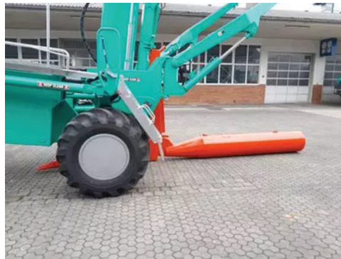
Laying steel pipes using the torpedo plow method
