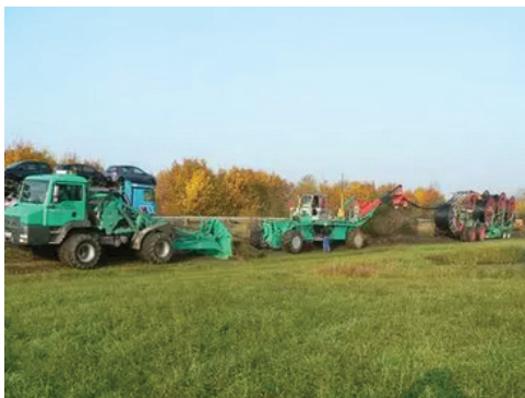
Laying of power cable
