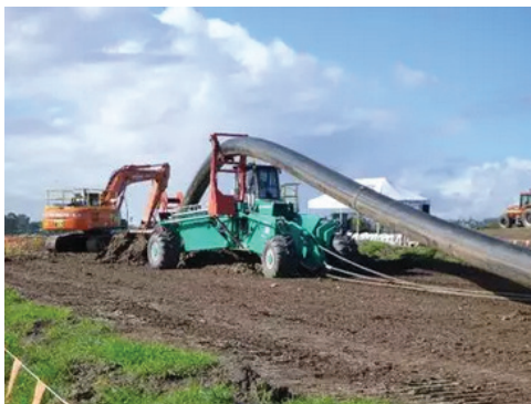
Laying of gas- and waterpipes
