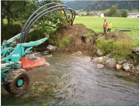
Laying pipes through watercourses
