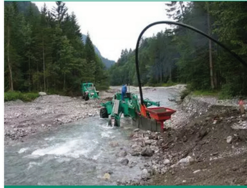
Laying system on rocky ground
