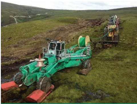
Laying system in mud and bog areas
